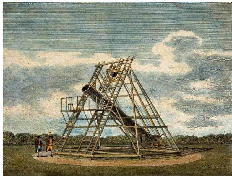
Figure 22 William Herschel's 40-foot (12 m) reflector
